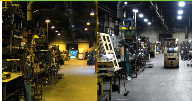
Eck Industries, Inc.'s manufacturing facility before the lighting retrofit.
