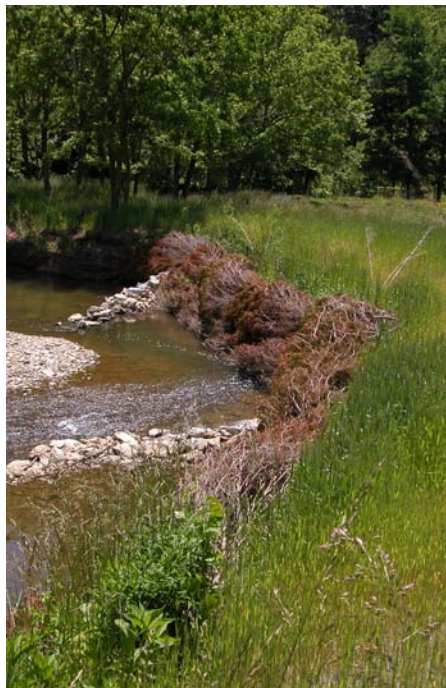
Protected and restored streambank with in-stream structures.
