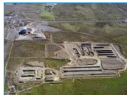
An aerial view of the F-Area at the Hanford Site in Washington State shows a wide range of waste sites during mid-cleanup activities.
