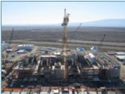
The High-Level Waste Vitrification Facility, shown here, is one of four major facilities under construction as part of the Hanford Tank Waste Treatment and Immobilization Plant, which is being built at the Hanford Site in Washington State. The plant will treat radioactive and hazardous waste currently stored in 177 underground tanks.
