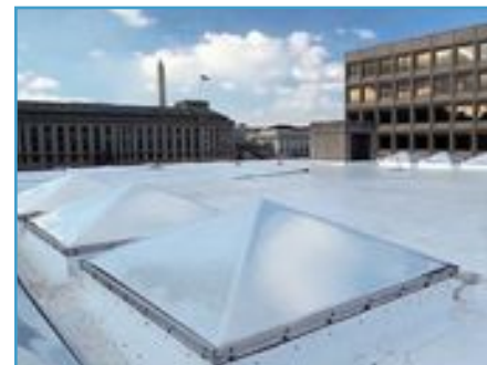
Cool roofs—as shown here on the DOE Headquarters building—use lighter-colored roofing surfaces or special coatings to reflect more of the sun's heat, helping to improve building efficiency, reduce cooling costs, and offset carbon emissions.
