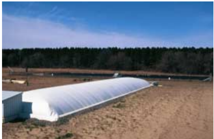
Anaerobic plug-flow digester. Haubenschild Farms, Inc.
