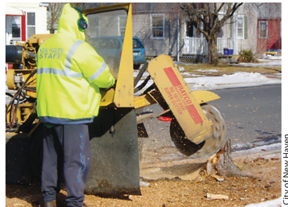
Figure 8: Tree-Stump Removal
