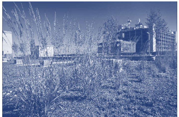
The Morgan mail processing facility in midtown Manhattan features New York City's largest green roof.
