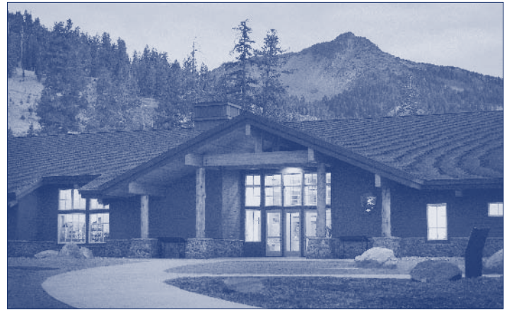
Opened in September 2008, the Kohm Yah-mah-nee Visitor Center in Lassen Volcanic National Park is a LEED Platinum facility.
