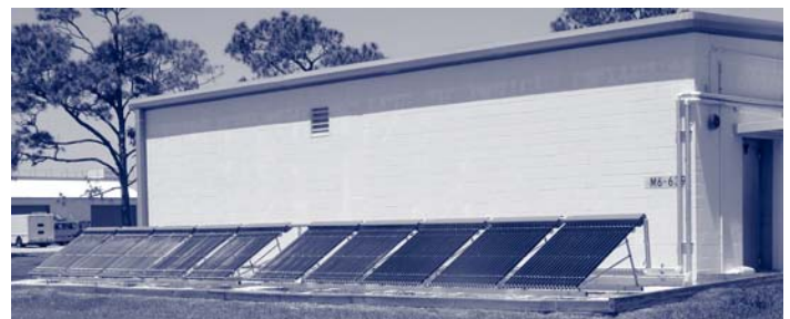
Solar heating system at Kennedy Space Center’s film storage building.
