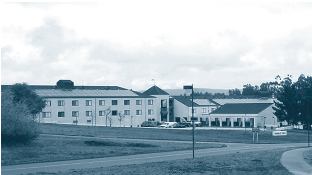
Attractive roof-mounted PV systems can be seen on the sloped roof of the Horsley Hall Barracks, Petaluma, CA.
