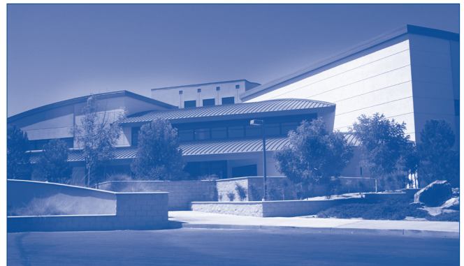
A thermal energy storage plant houses six large ice tanks that help cool the 95th Air Base Wing Consolidated Support Facility shown here.
