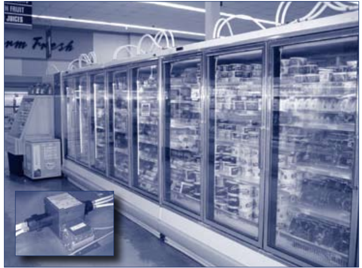
Fiber optic lighting installed in commissary reach-in freezer display cases. Photos by Steven Parker, PNNL.
