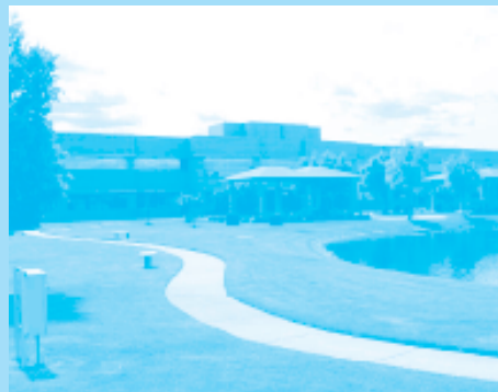
DOE’s Bechtel Hanford Headquarters in Richland, Washington, uses an array of energy- and water-saving technologies.
