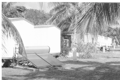
The second solar water heating system installed at AUTEC.
