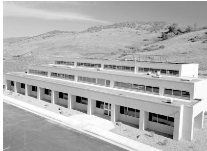
The Thermal Test Facility is an energy-efficient, state-of-the-art laboratory in which NREL researchers and their Federal and private-sector partners can investigate and develop advanced building components and systems.
