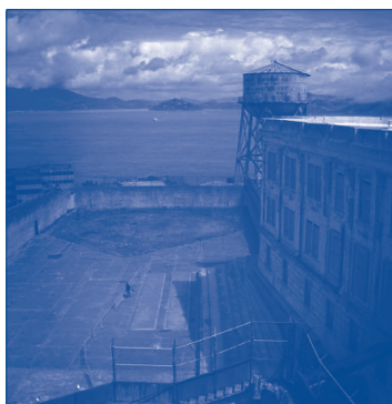
Roof of old cellblock and possible PV installation location at Alcatraz
