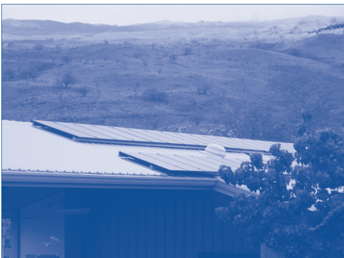
Solar array at Pu'ukohola Heiau National Historic Site Building
