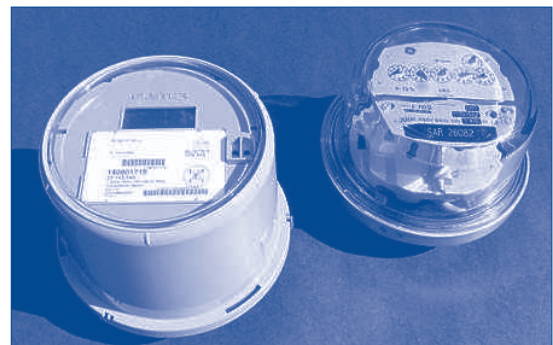
"Smart" (left) versus standard meter (right)
