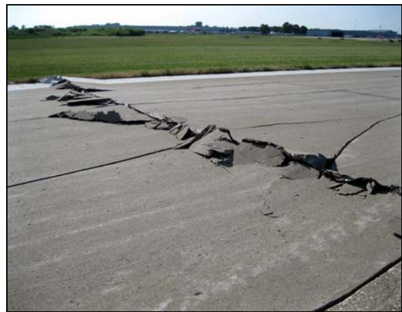
Pavement Buckling
