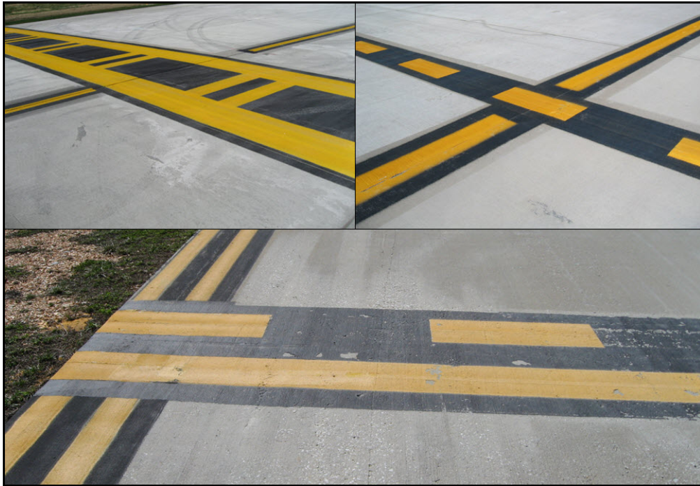
Pattern B (ILS Hold Position), Pattern C (Hold Position for Taxiway/Taxiway intersections) and non-movement area marking.
