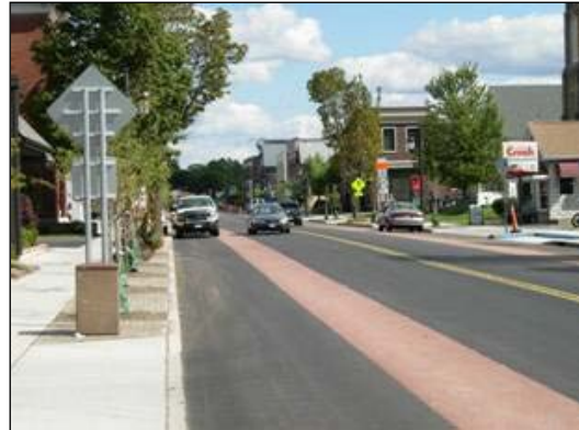
Hamburg's roundabouts and road diet improved capacity, safety, and business access. The top picture shows a roundabout with raised truck apron and central landscaping. At bottom, a colored buffer zone separates parking from narrower travel lanes.
