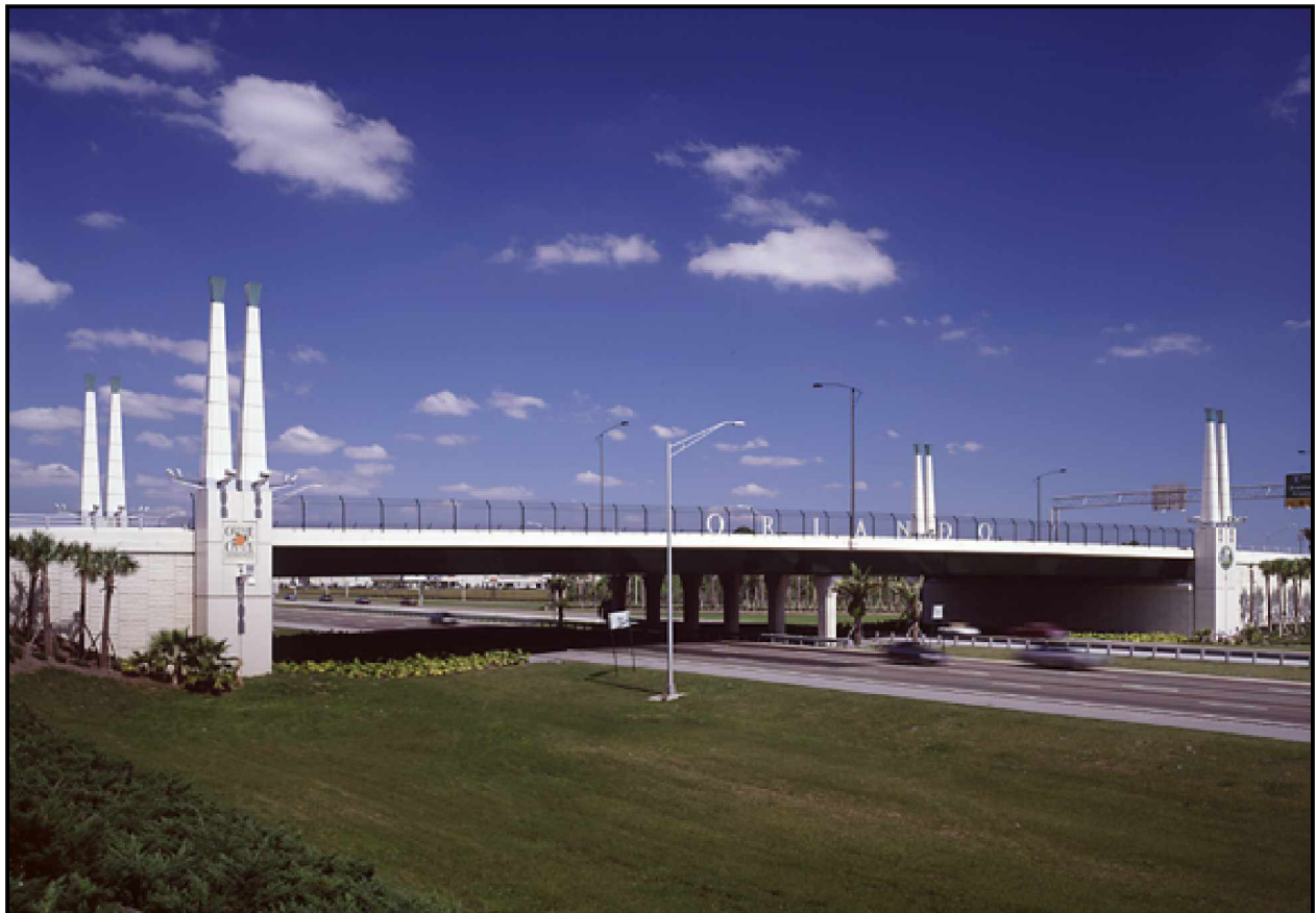
Exhibit 3.39 - Conroy Road Bridge over I-4 in Orlando, Florida
