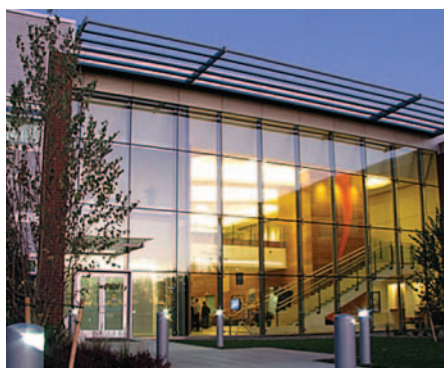
Figure 27. PNNL CSF/BSF building entry area. Photo courtesy of PNNL
