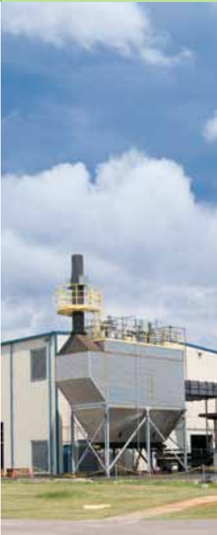
U.S. Department of Energy Savannah River Biomass Steam Plant Savannah, GA
