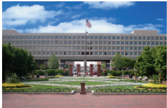
The Department of Energy's Forrestal Headquarters building in Washington, DC, achieved a score of 88 on the ENERGY STAR rating scale, outperforming almost 90 percent of office buildings nationwide.
