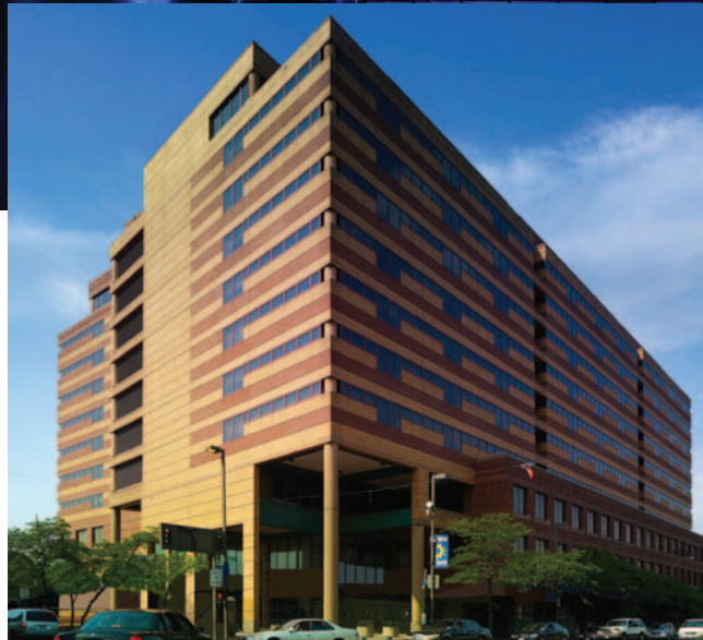
The Joseph P. Addabbo Federal Building in Jamaica, NY, replaced the entire building's chiller plant and is currently completing the final phase of related upgrades to its building control system.
