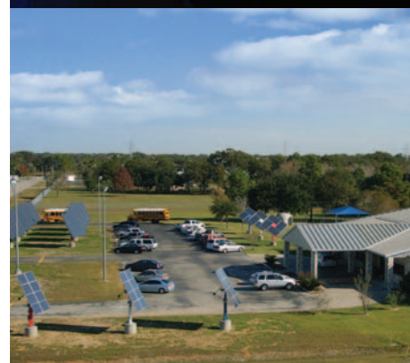
Johnson Space Center Child Care Center, Houston, TX. To help reduce conventional energy demand and greenhouse gas emissions, NASA's Johnson Space Center constructed a Multi-Platform Renewable Energy System at its on-site Child Care Center.
