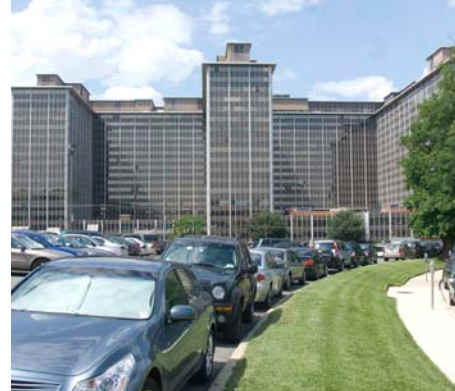
The HHS Parklawn Building Program Support Center, Rockville, MD, installed high efficiency chillers, upgraded boiler components, applied solar film to 8,740 windows, and replaced 55,679 T-12 lamps with more efficient T-8 lamps.
