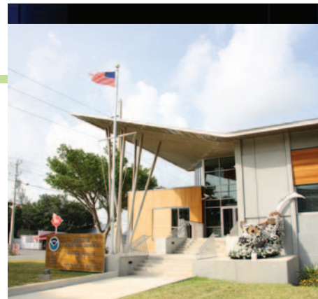
The National Weather Service's Weather Forecast Office (WFO) in Key West, FL, is one of 122 WFO's that monitor and predict weather patterns to help protect the nation, and is the second to obtain a LEED Silver rating.
