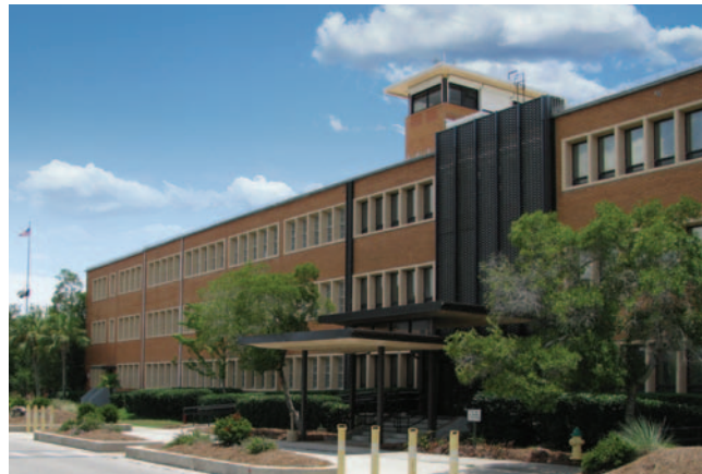
The Naval Surface Warfare Center Panama City, FL, with technical assistance from the host command Public Works Department and the Naval Support Activity Panama City, retrofitted a 400-ton state-of-the-art chiller compressor system into existing chillers.
