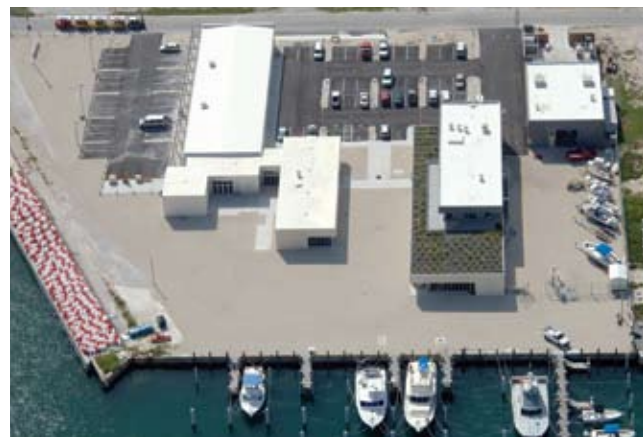
NOAA's Dr. Nancy Foster Florida Keys Environmental Complex includes a green roof, sustainable building materials, and energy efficient technologies that reduce energy use by 30 percent.
