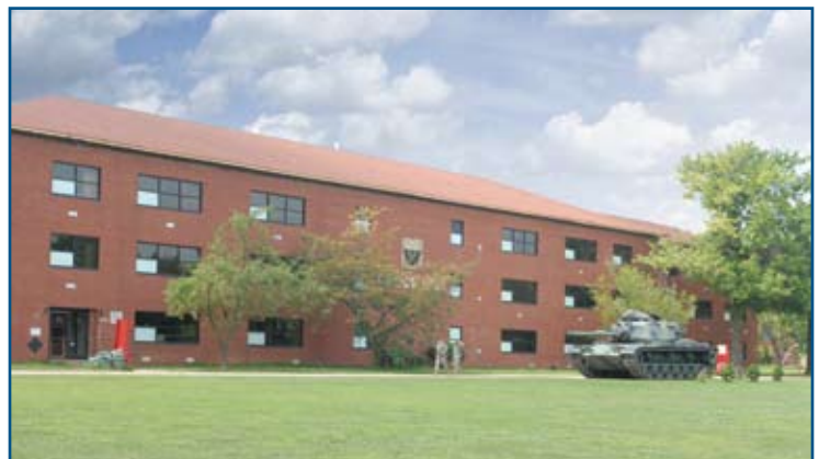
The Fort Knox Disney Barracks Area is made up of 38 buildings that comprise more than 800,000 square feet. UESCs helped replace 70 percent of the existing HVAC system with geothermal heat pumps and new ventilation systems to save more than $800,000 each year.
