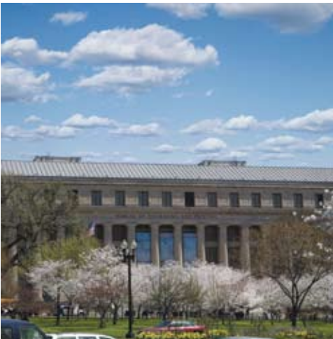
The U. S. Department of the Treasury's Bureau of Engraving and Printing facility in Washington, D.C. implemented an energy reduction strategy to monitor and control 86 air handling units via Web-based Intranet.
