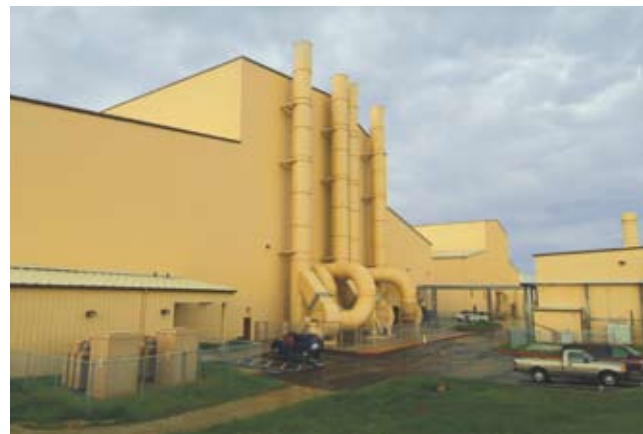
The Robins Air Force Base Large Aircraft Corrosion Control Paint and Depaint Hangar uses the first air recirculation system in the Air Force, and saves $2 million each year.
