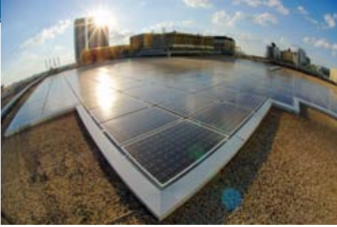
The Harold Washington Social Security Center in Chicago, Illinois, used UESCs and ESPCs to reduce energy use by 20 percent and save 2 million gallons of water each year.
