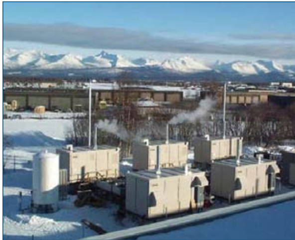
The USPS in Anchorage, Alaska, uses power generated by highly efficient, low-emission fuel cells.
