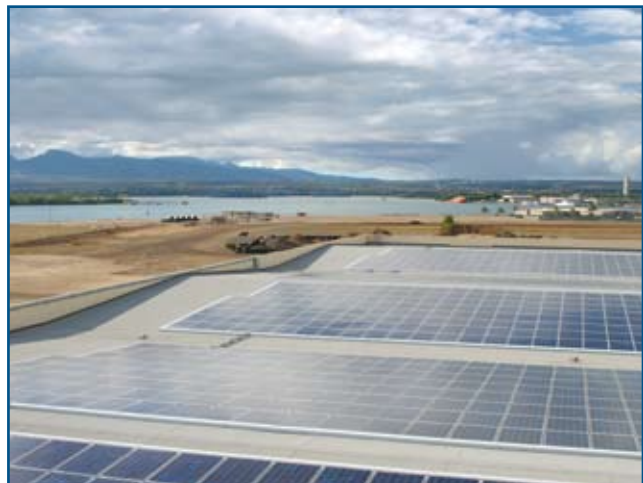
Building 54, Pearl Harbor Naval Facilities Engineering Command, HI, a historic World War II aircraft hangar, now has a 309-kilowatt photovoltaic array on its roof.
