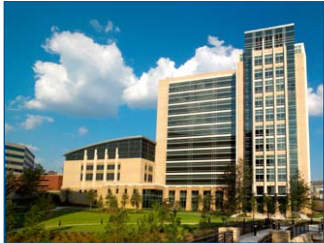
The Edward R. Roybal Campus, Centers for Disease Control and Prevention, Atlanta, GA, includes three new sustainable buildings, a central utility plant, and a self-sustaining green space.
