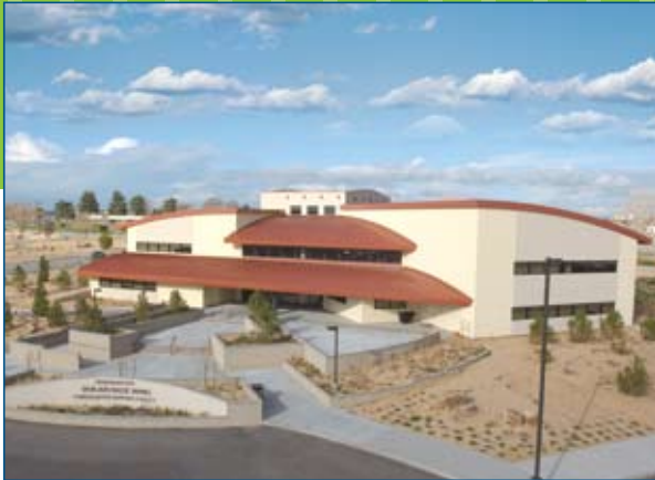
The Edwards Air Force Base Consolidated Support Facility incorporates a unique cooling system to meet daily demands through off-peak, night-time generation of thermal energy in ice banks.
