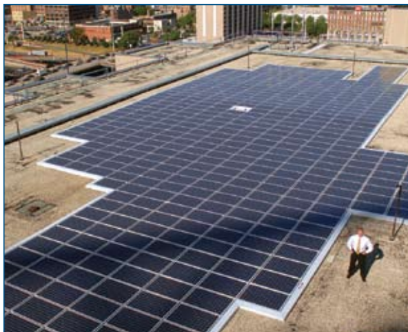
The 100 kilowatt solar electric system at the Harold Washington Social Security Center, Chicago, IL, generates enough electricity to offset peak power demands.
