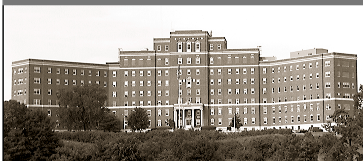
The Veteran's Administration Medical Center at Providence, Rhode Island will benefit from a FEMP SAVEnergy audit.
