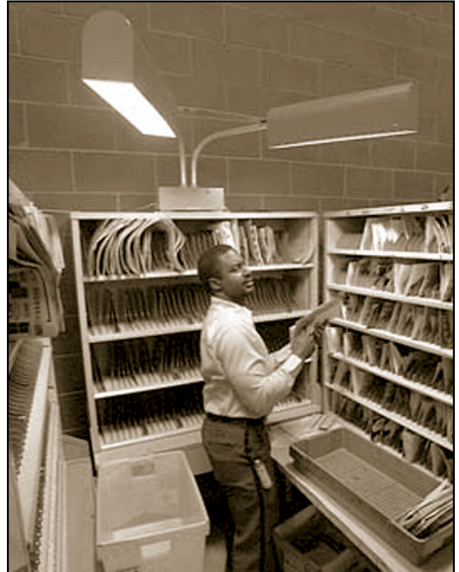
Improved task lighting at the Rodeo, CA Post Office has increased worker productivity while reducing energy costs by 30%.
