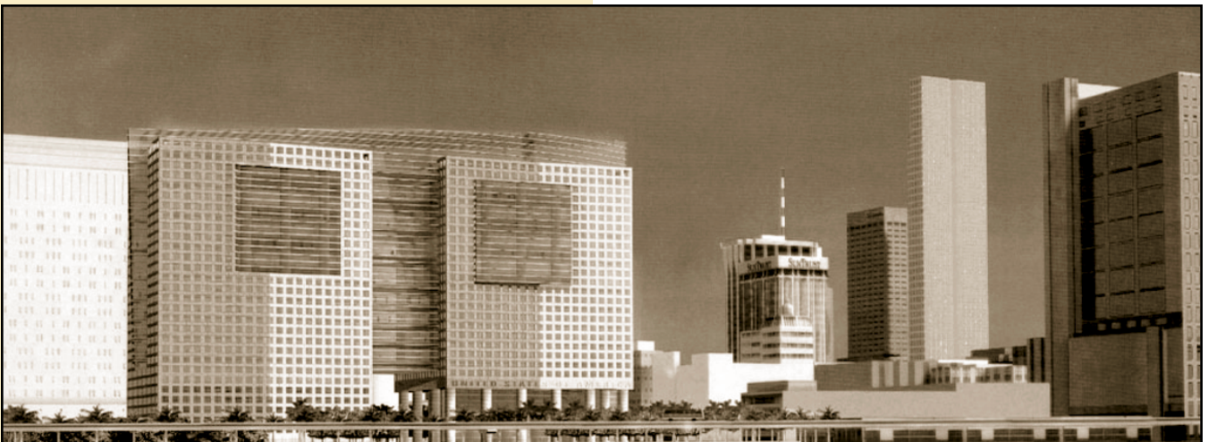
The Miami Courthouse design employs a curtain wall with large expanses of glass and high-performance window glazing.
