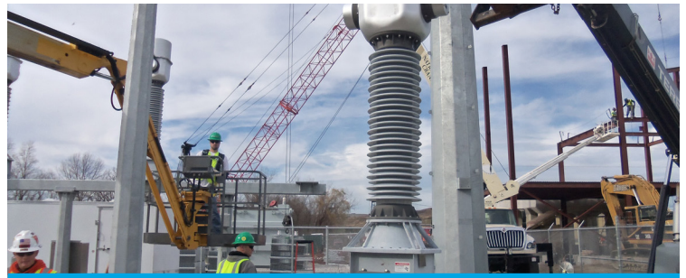
Installing equipment in the Johnston, Rhode Island facility's switchyards.
