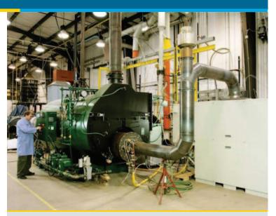
The FlexCHP-65 system consists of Johnston Boiler Company 100-horsepower firetube boiler, GTI-developed supplemental Ultra-Low-NO\_x burner, and Capstone C65 microturbine.
