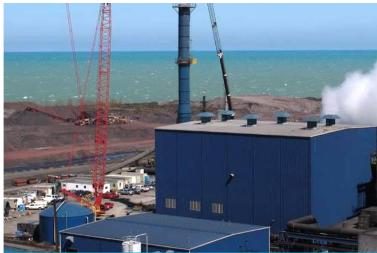
ArcelorMittal USA blast furnace gas flare capture project under construction in 2012.
