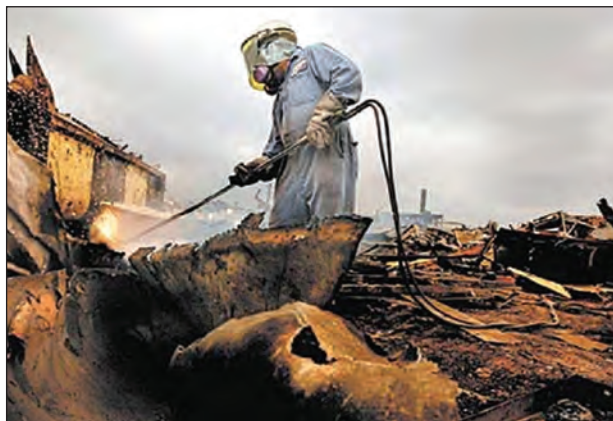
Worker torch-cutting scrap metal from vessel.
