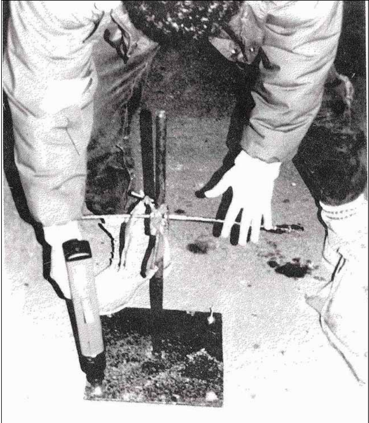
Figure 5. Setting an Erected Stringline
