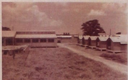
COMPARE THESE NEAT, clean houses at the FSA camp with the shack across the page.
