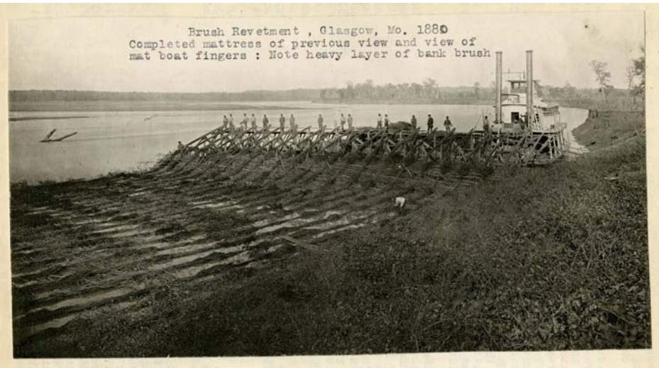
Original caption: Brush revetment, Glasgow, MO circa 1880. Completed mattress of previous view and view of mat boat fingers; note heavy layer of bank brush. RG 77, Records of the U.S. Army Corps of Engineers.
