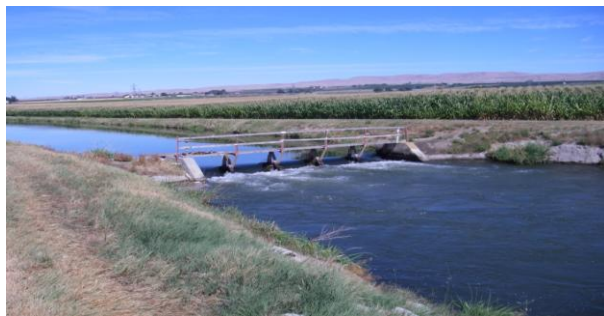
Figure 1. Picture of a manual check structure used to control water elevation are dangerous to adjust and labor intensive.
