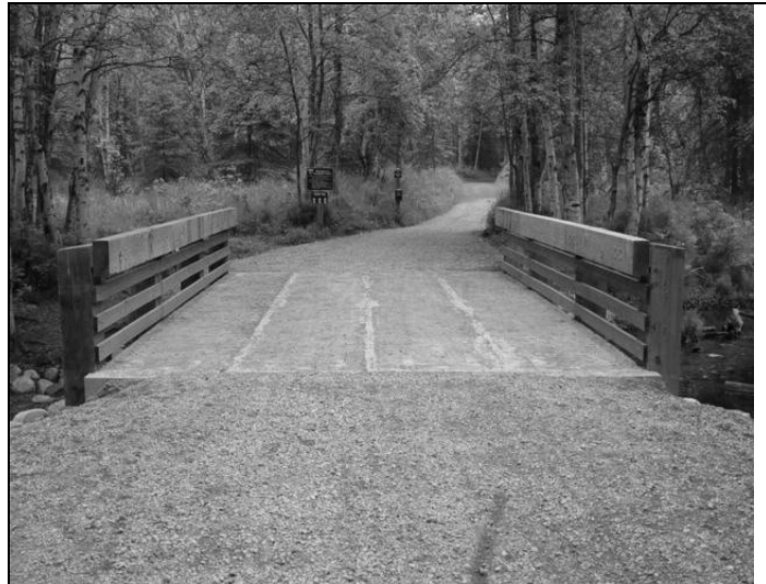
Little Campbell Creek Bridge located in Anchorage, Alaska, completed in 2008.
