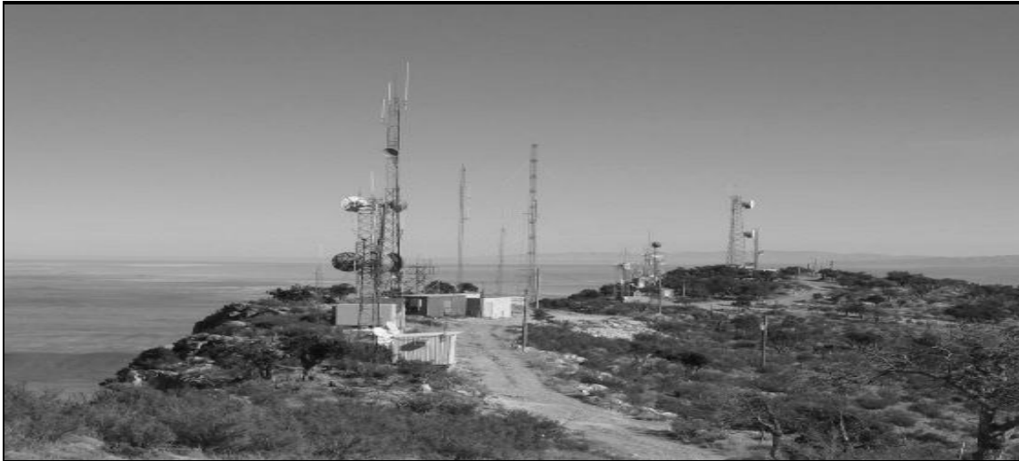
Site Inspection: Caballo Communication Site Las Cruces Field Office
