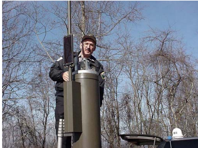
Figure F- 5. Working on a gage.
