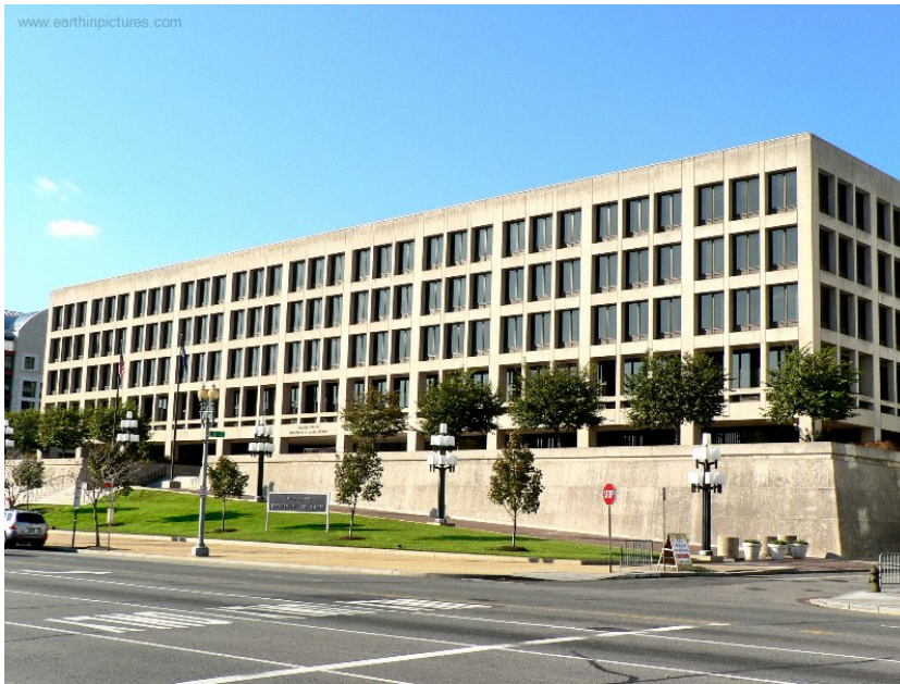
Figure 1. Frances Perkins Building exterior view from Constitution Avenue.
