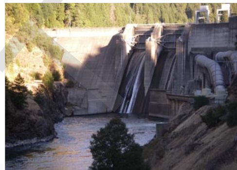
Dam impeding fish passage.
