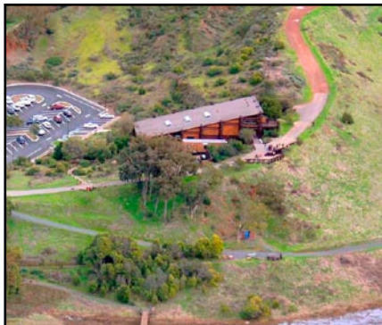
The project will renovate the 9,022 square foot 1970s vintage headquarters office at San Francisco Bay NWR. Modifications include a new shingle roof, thermal-pane low-e windows and doors, expansive foam wall and ceiling insulation, high efficiency lights, solar-thermal hot water, and other modifications. (photo: USFWS)
