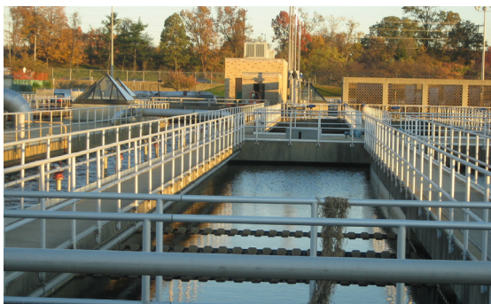
The Blue Plains Wastewater Treatment Plant serves the Washington, DC, metropolitan area and is the largest wastewater treatment facility in the Chesapeake Bay watershed (EPA OIG photo).
