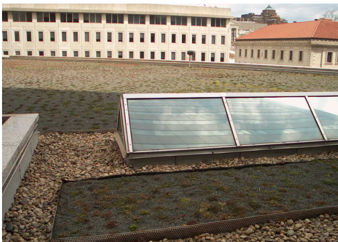
With the help of an EPA grant, a bank installed a “green roof” on one of its buildings in Richmond, Virginia. Among its many benefits, the green roof reduces polluted stormwater runoff. (EPA OIG photo).
