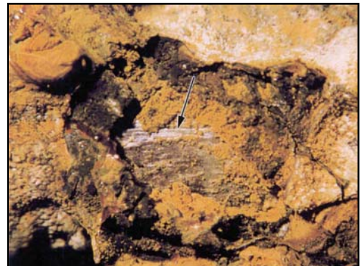
Figure 23. Champlain II #17 iron rod. Arrow points to corrosion in the longitudinal direction under the scale. Magnification 6.5x.
