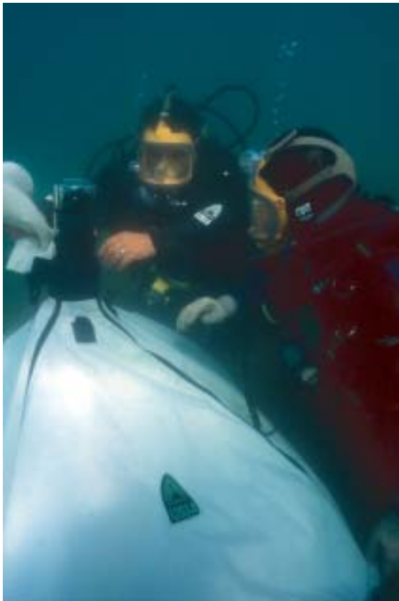
Figure 11. Oil catchment device deployed on hatch to starboard of Barbette No. 4.
