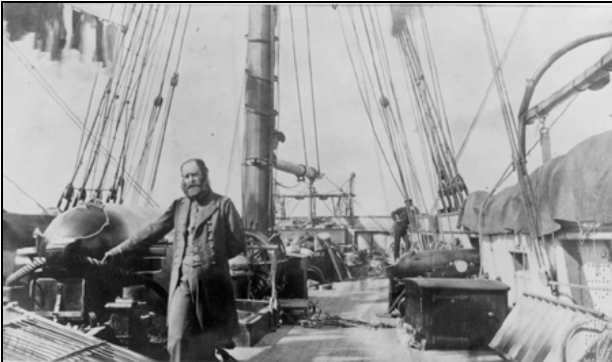
Figure 7. Historic photograph illustrating a Fawcett, Preston & Co. 32-pounder, an ordnance chest and the tangent sight on the breech of the stern pivot gun of the CSS Alabama .
