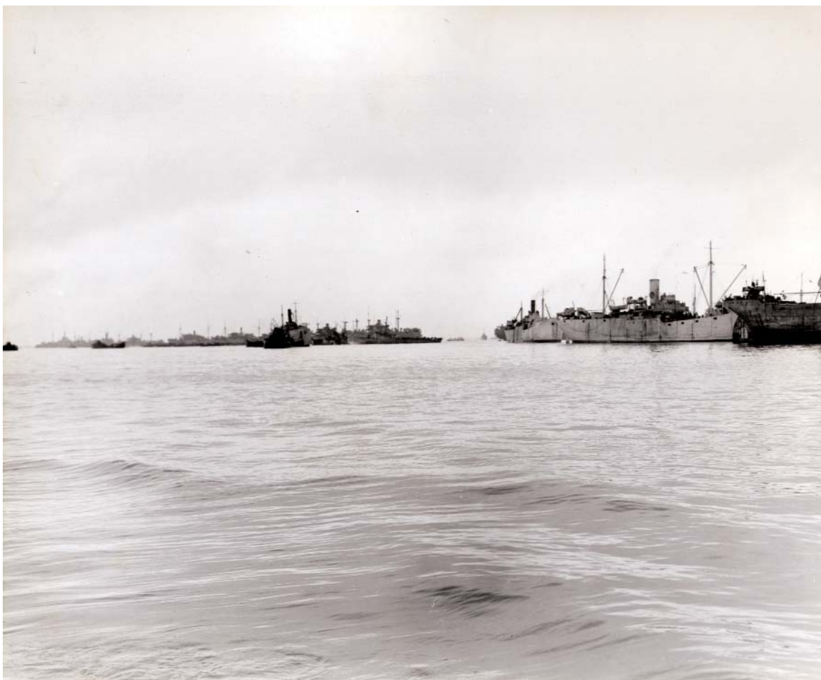
Above: The Gooseberry line of sunken ships (National Archives Photograph No. 80-G-284124).
