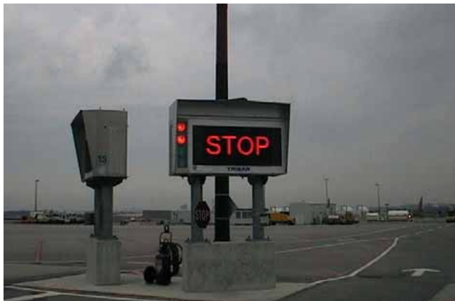
Figure 3-5(b). Electronic message board informing the pilot the aircraft has reached the stop point of the deicing pad
