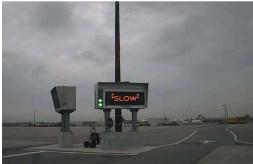
Figure 3-5(a). Electronic message board instructing the pilot to continue forward to the stop point of the deicing pad
