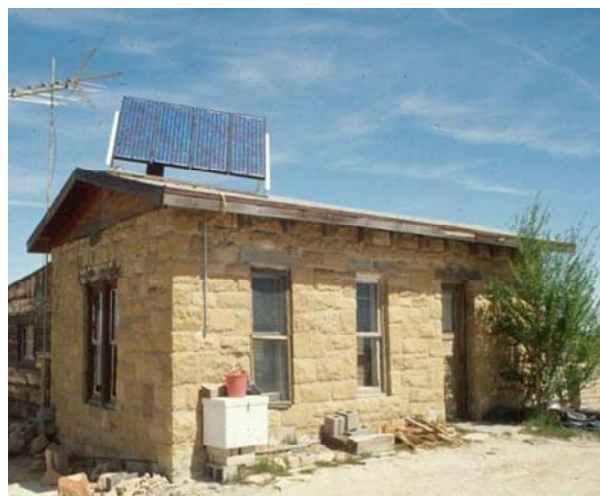
Figure 4. The 240 watt model unit deployed in Hotevilla, Arizona, is owned and operated by a former NativeSUN employee. It is sufficient for a small direct current (DC) television, a radio, and two 22 watt DC fluorescent circular lights.
