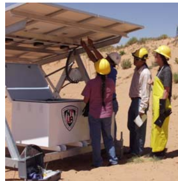
Figure 5 shows NTUA electrician, Vircynthia Charley, working in the cramped quarters of the 640 Watt battery box. In Figure 6, NTUA's Larry Ahasteen, shows Sandia student interns the improved working conditions under the Phase I 880 Watt array.
