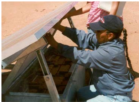
Figure 5 shows NTUA electrician, Vircynthia Charley, working in the cramped quarters of the 640 Watt battery box. In Figure 6, NTUA's Larry Ahasteen, shows Sandia student interns the improved working conditions under the Phase I 880 Watt array.
