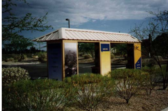
Figure 5-18. Public charging station with informational graphic panels.
