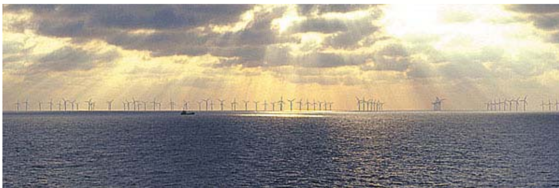
Figure I-6. Nysted Wind Farm, 14-20 kilometers (km) offshore Denmark, the North Sea (Source: DONG Energy 6 )
