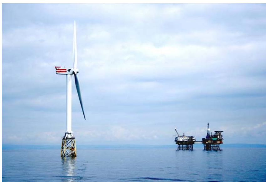
Figure I-1. RePower Systems 5M, The World’s Largest Wind Turbine (5-MW, 126m tall, 45m depth)
