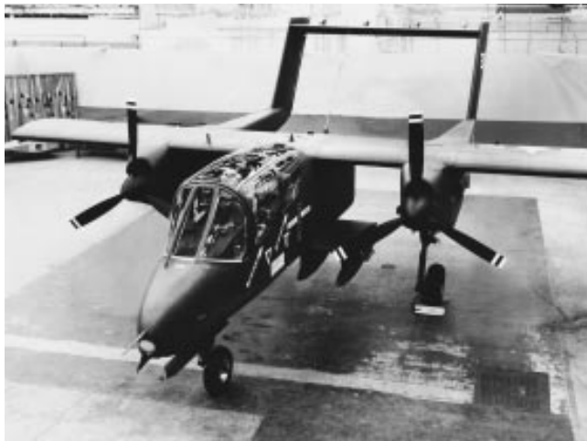
A full-scale mock-up of the OV-10 at the North American factor, circa mid-1960s.
