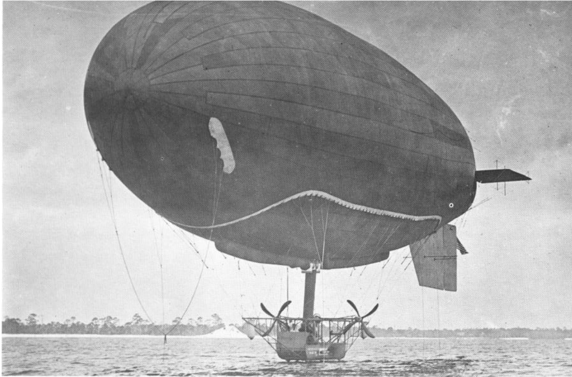
Photographed on April 27, 1917, the Navy's first nonrigid airship, DN-1, maneuvers on the water at Pensacola, Fla. Due to manufacturing problems and poor engines, it could barely get airborne. AN 8293
