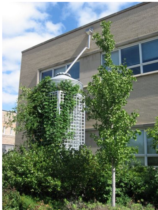
Figure 5. Rain water cistern.
