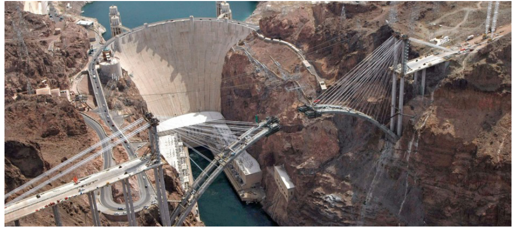
Figure 1. The Hoover Dam (background) used 3.25 million cubic yards of concrete to build, while the still-under-construction Mike O’Callaghan–Pat Tillman Memorial Bridge (foreground) will require a further 32,000 cubic yards of concrete.
